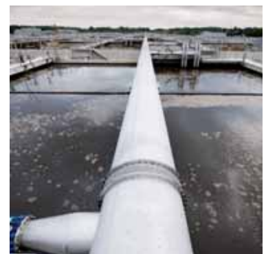
Aeration of the wastewater using Siemens' Sitrans process instruments. Credit: Siemens.
