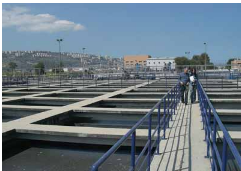
Sedimentation at the Haifa wastewater treatment plant. Credit: Dahlem Consulting Engineers, Germany.
