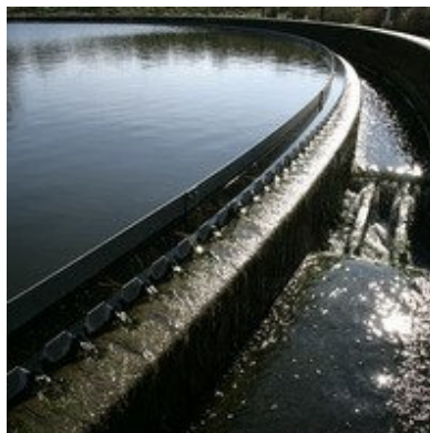
Wastewater treatment plant: discharge of purified wastewater from clarifier
