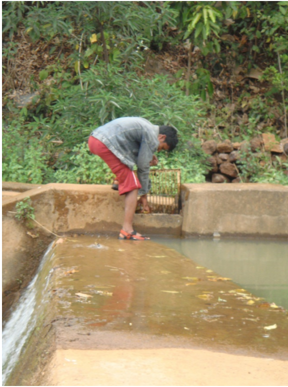
Figure 2.4: Cleaning the intake channel in Putsil.
