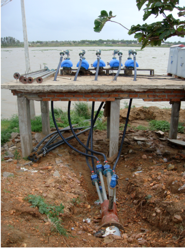
Figure 3.3: Lift irrigation pumps installed along Tungabhadra River at Bennur.
