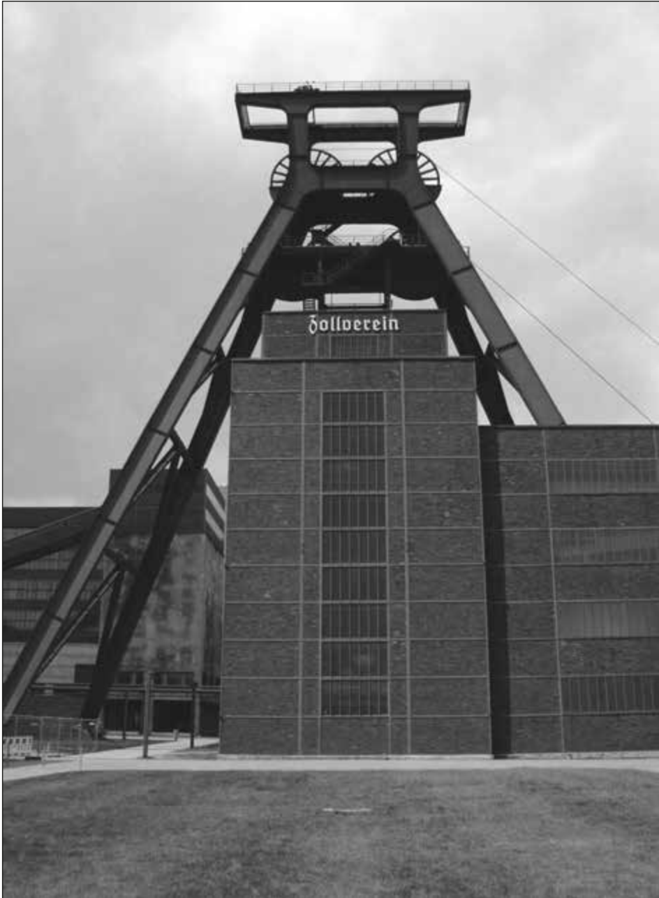
Fig. 8.1 The iconic steel hoisting frame over Zollverein's central Shaft XII. This hoisting frame was used to raise and lower conveyances within the mine shaft to transport coal, which was later sent to the coal washing plant where it was separated from rocks and other unwanted material. Although the mine ceased production in the 1986, the hoist is still used to pump water out of the empty mine shafts. Picture by the author (2014).
