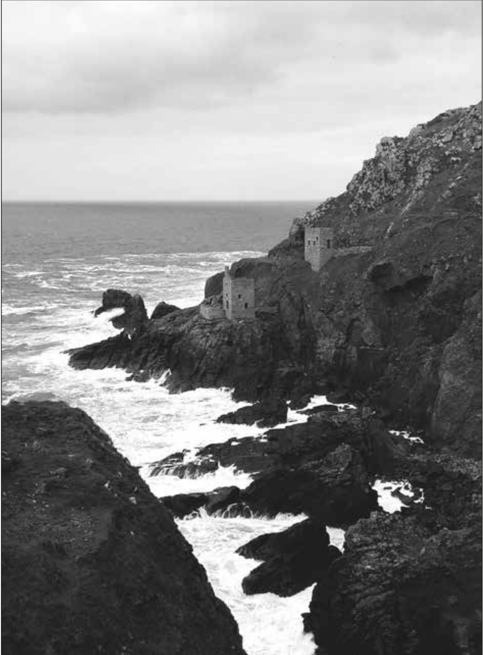
Fig. 9.2 The Crown engine houses at Botallack mine, Saint Just mining district. These engine houses were constructed in the 1860s to drain mine shafts that reached almost 400 meters under the Atlantic Ocean. In the 1980s the property was acquired by the Botallack Trust and is owned by the National Trust since 2002. Picture by the author (2015).
