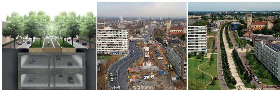
Figure 2. Left: Schematic overview of the tunnel and the Green Carpet on top of it; Middle: Highway A2 crossing the city of Maastricht, during construction of the tunnel; Right: Green Carpet after the opening of the tunnel. Source: Projectbureau A2 Maastricht.
