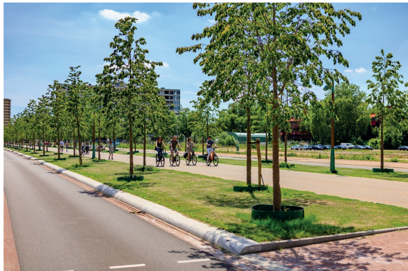
Figure S1.b. Picture of the Green Carpet showing the profile consisting of a semi-paved middle path, adjacent one-way streets, and green strips separating them. Source: Projectbureau A2 Maastricht/ Fred Berghmans.
