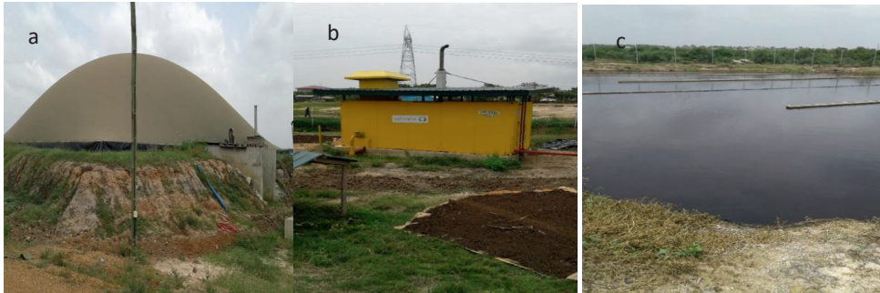
Fig. 7 (a) The Safisana fixed-dome biogas plant, Ashaiman, Accra, September 2017, (b) The CHP at the Safisana Ashaiman site, September 2017; (c) Waste stabilisation pond with baffles at the Ashaiman site for treatment of liquid waste from the drying beds, September 2017
