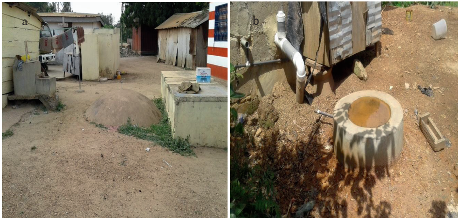
Fig. 5 (a) Remains of a fixed-dome digester at Appolonia, Accra, October 2017; (b) fixed-dome digester not connected to a kitchen at Cape Coast, Central region, October 2017
